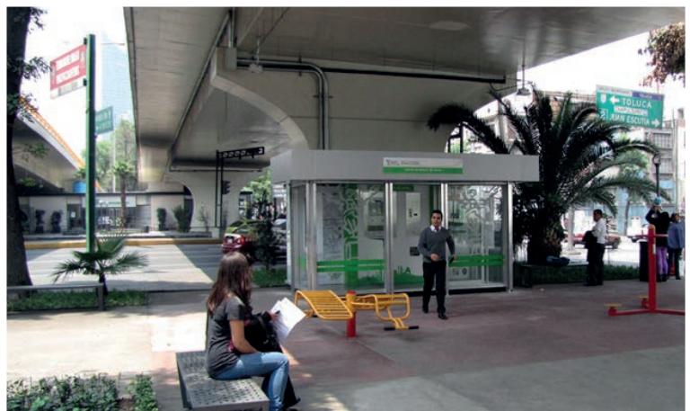
Bajos Puentes Underpass Program (2013), Mexico City MX
